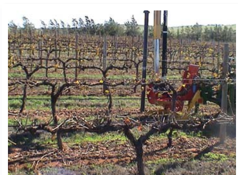
Hammer installation in progress. APR Vineyard Posts have been field tested for hammer, vibration hammered and water drilling installation.
